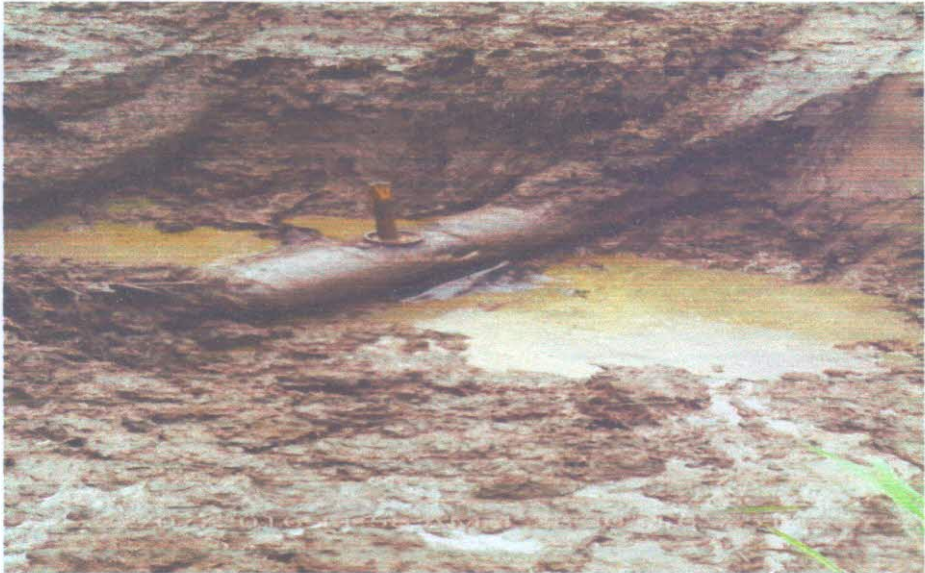
POINT DURING REPAIR SHOWN: fig2
